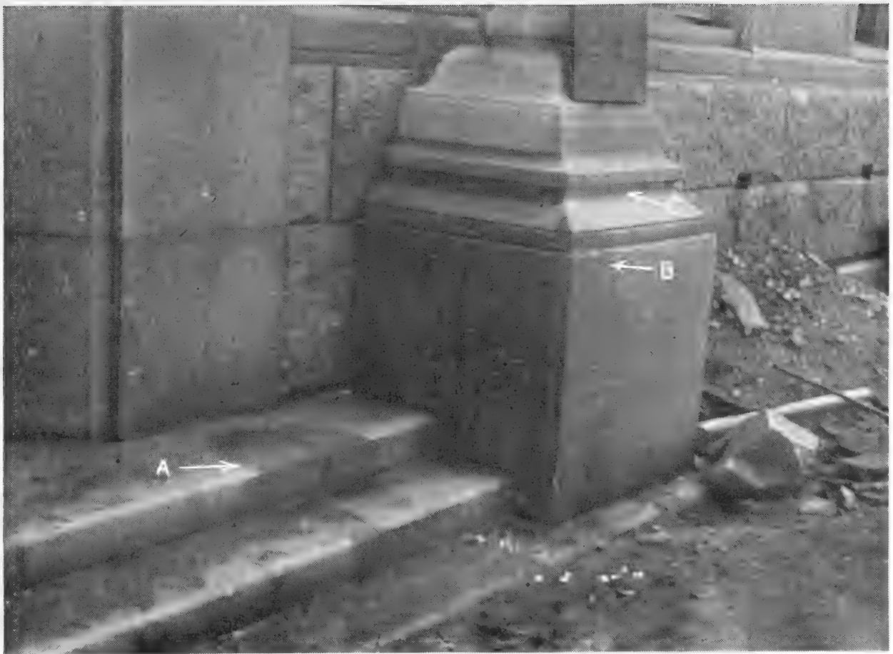
Photo No. 21. HIROSHIMA. Roughening of polished granite by "flash" heat effect at 200 yds. from the centre of damage. The polish remains only where shielded by (a) a man seated on the steps, (b) a man leaning against the corner of the plinth adjoining the steps and (c) in the "shadows" of the plinth mouldings. See paragraph 49.
